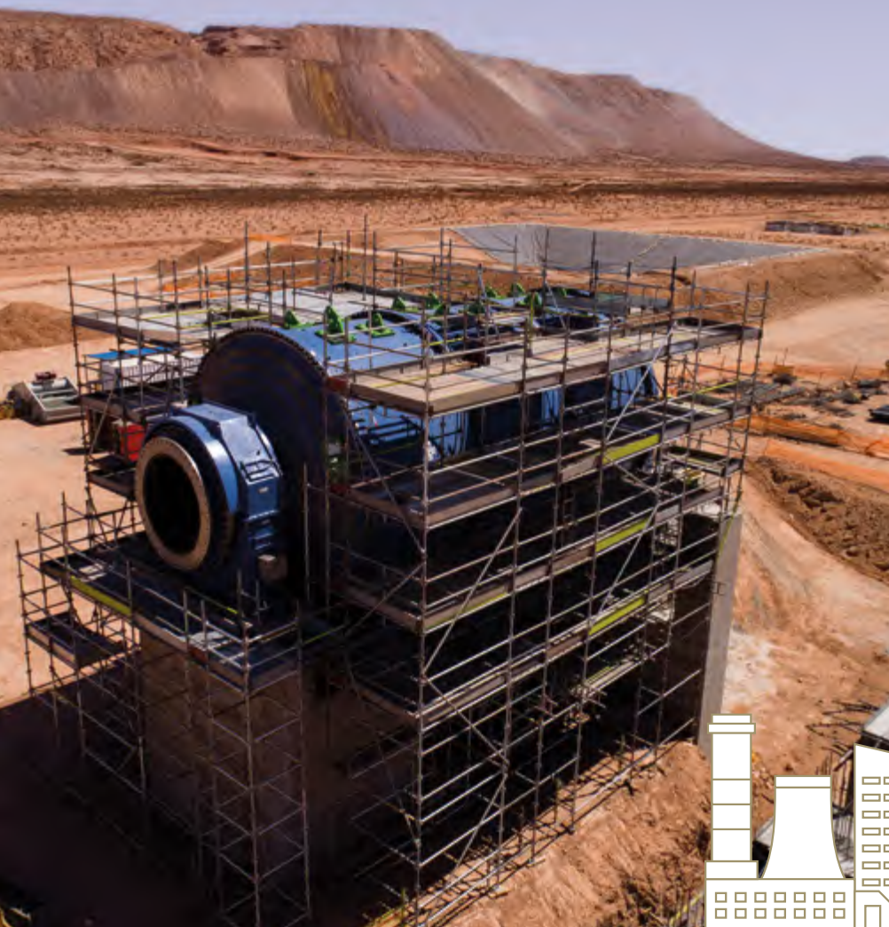
Erection of ball mill shells, bearing housing and motor.
