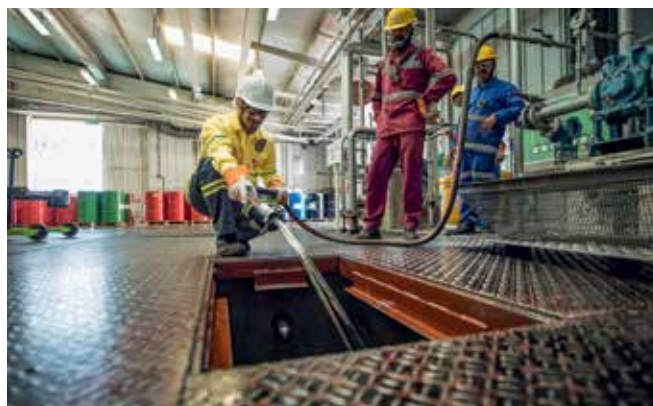
Shell lubricant plant, Oman.
