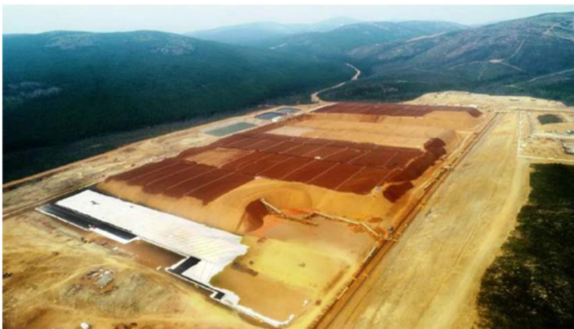
Figure 4-10: Gross Dynamic HLF Looking West (July 2019)
